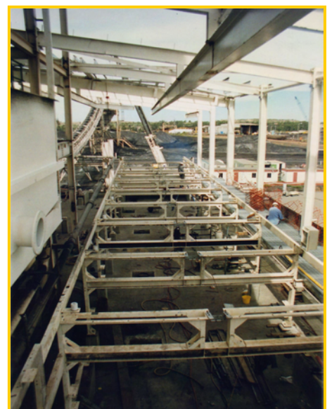
110 square belt filter bed during construction.
